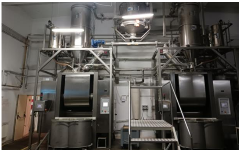
Fig. 7 Dosing line for raw materials
